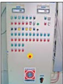
All systems can be supplied with fully automatic control with monitoring of the whole paint and drying process.
